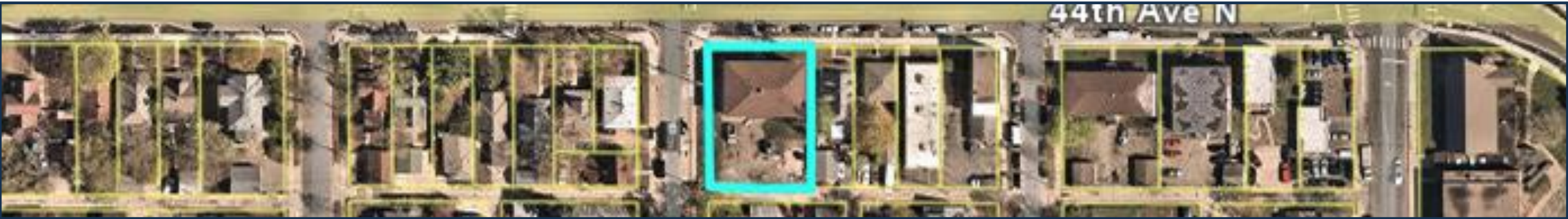
The property as we found it — half-vacant, overgrown, unpaved parking
